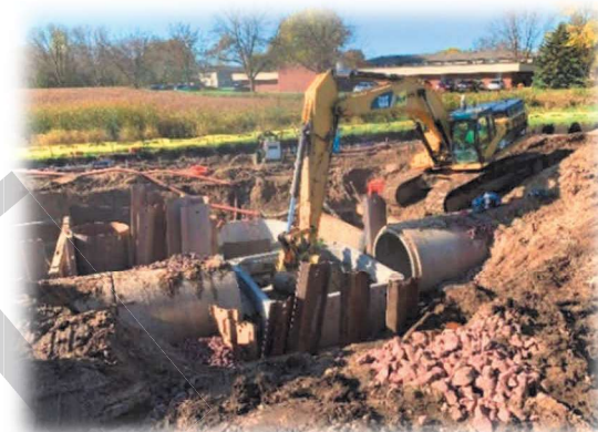
Figure E-7: Stormwater improvements on a tributary to South Creek
