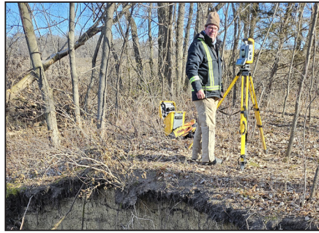
Left: Civil engineering technician Brian Jacobs surveyed a large gully along Butterfield Creek in Watonwan County. A rock chute was later installed at the site to allow water to flow in and out of the creek during high water events. Middle: South Central TSA senior civil engineering technician Greg Schemmel surveyed the site of an embankment failure in Sibley County using a total station, a surveying instrument that measures distances, angles and coordinates. Right: South Central TSA engineer Ryan Jones assessed erosion in a ravine channel downstream from a potential project site in Sibley County.
