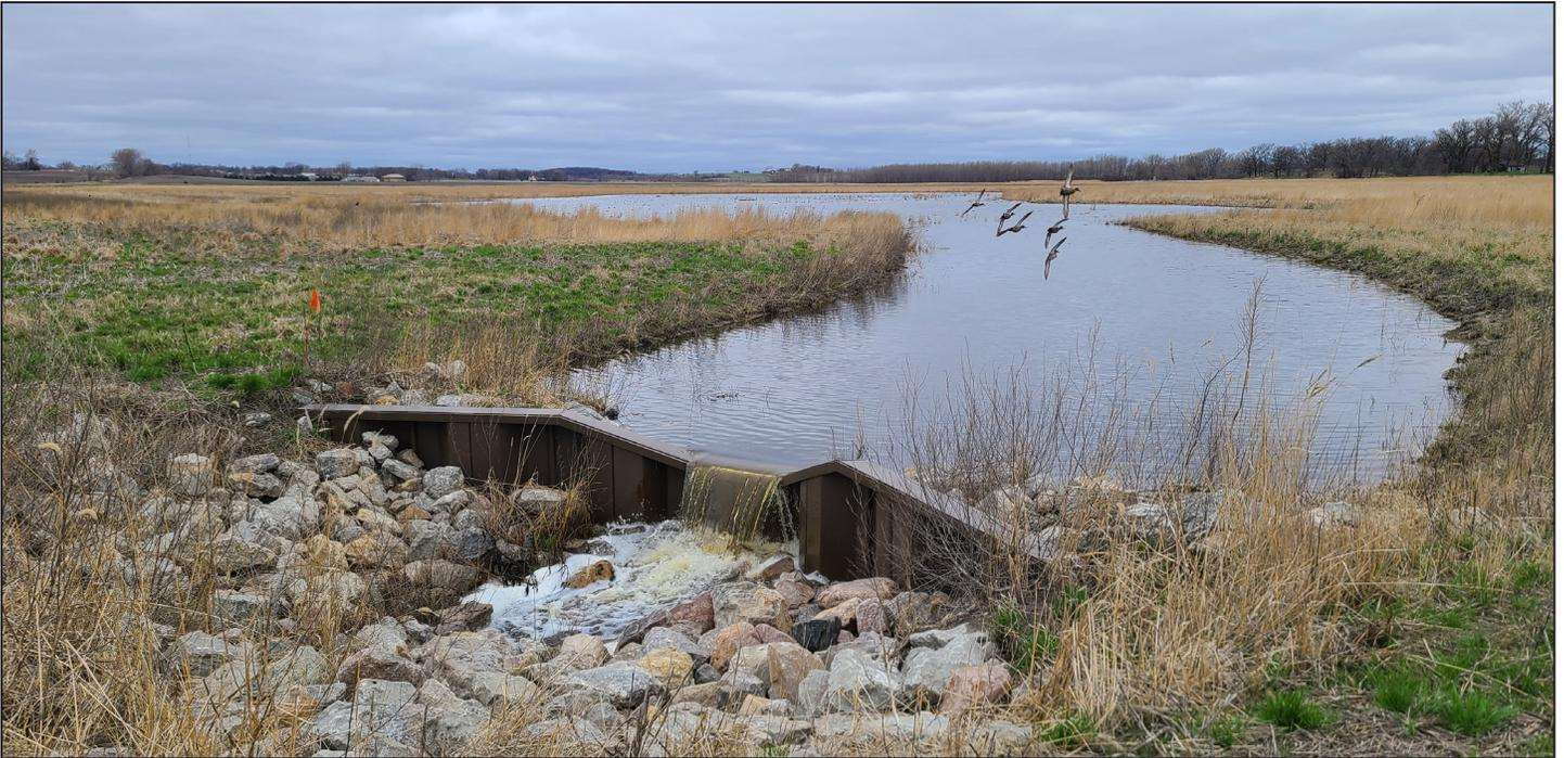
An outlet structure was installed as part of a wetland restoration on this MN CREP easement in Freeborn County. Restoring the wetland reduced pressure on the county ditch system while providing water storage and wildlife habitat. **Photo Credit:** BWSR
