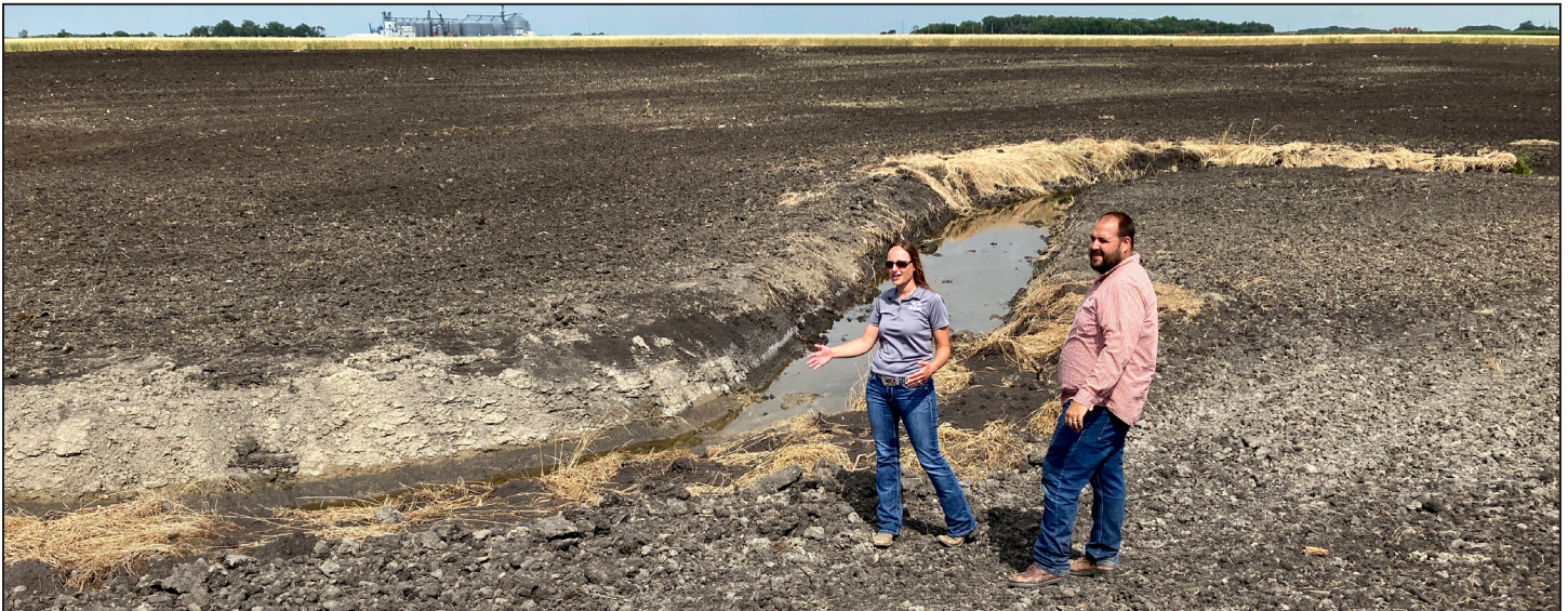
Melton and Quast discussed progress of the Whiskey Creek project on Aug. 2, 2022, as they walked along a newly re-meandered stream segment near Breckenridge. Phase 2 of a planned $7 million, 20-mile-long Whiskey Creek restoration was completed in 2022. Related upland practices bring the total cost to $9.9 million. Clean Water Fund grants from BWSR and a National Water Quality Initiative award from NRCS are among the funding sources.
