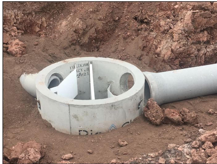
Above: A hydrodynamic separator was installed to collect sediment from stormwater pipes before it’s discharged into Skunk Creek. Below left: A health advisory sign posted at Agate Bay indicated high levels of E. coli bacteria. The Minnesota Department of Health conducts weekly Lake Superior beach monitoring from Memorial Day to Labor Day. Below right: Stormwater drains into Burlington Bay. Photo Credits: Lake County SWCD
