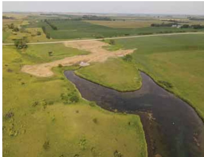
Two grade stabilization structures share a berm in the northwest side of Del Clark Lake. The two structures, plus a roadside retention embankment near the south area of the lake, are estimated to capture a combined 667 tons of sediment each year.
