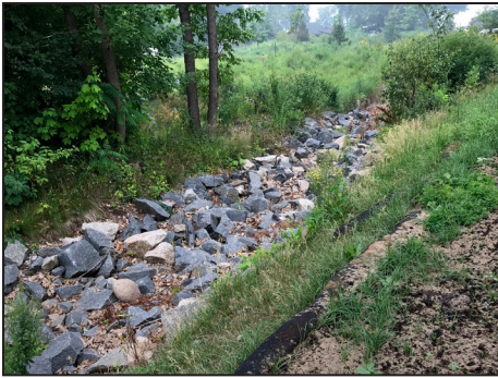
Above: A two-stage retention basin and iron-enhanced sand filter slow and treat runoff from a 30-acre drainage area in Deerwood, removing about 90% of the phosphorus. At the Summer Place on Serpent Lake, heavy rains had flooded some — but not all — of the 13 cabins. Getting all 13 to agree to the project generated conflict and negotiation because those unaffected by flooding didn't want to give up land. Below: From left: Barrick, Michels, Tichenor and Chamberlin discuss the targeted watershed project at the new outlet to the lake.
