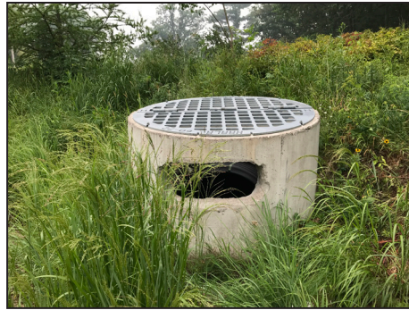
Above: A two-stage retention basin and iron-enhanced sand filter slow and treat runoff from a 30-acre drainage area in Deerwood, removing about 90% of the phosphorus. At the Summer Place on Serpent Lake, heavy rains had flooded some — but not all — of the 13 cabins. Getting all 13 to agree to the project generated conflict and negotiation because those unaffected by flooding didn't want to give up land. Below: From left: Barrick, Michels, Tichenor and Chamberlin discuss the targeted watershed project at the new outlet to the lake.
