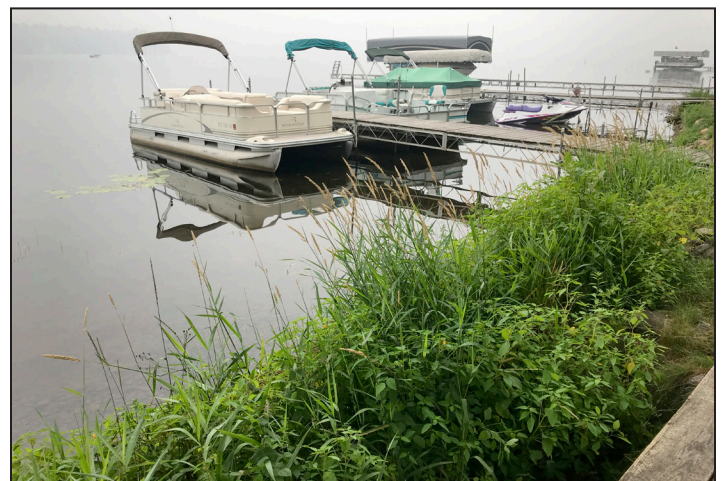
Top: A boardwalk covers the pipe that had sent untreated stormwater directly into Serpent Lake. Barrick stood in front of the outlet as she visited with Chamberlin, center, and Serpent Lake Association Board Member Jim Seletos.
