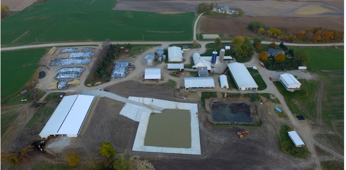
A manure pit and a roofed storage structure are part of a finished RCPP project in Rice County. Photo Credit: Nathan Pesta, DGA Engineering
