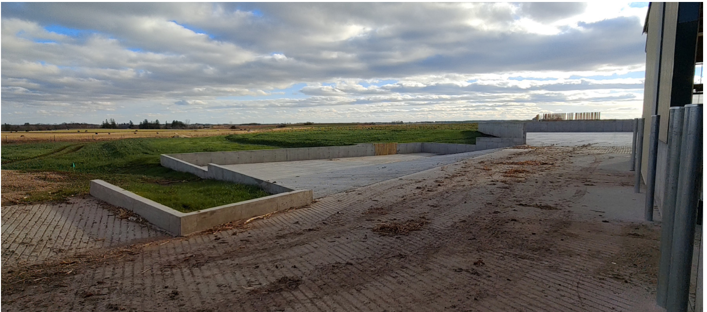
Manure is pushed from the barn to the storage area known as a stacking slab in this finished RCPP project in Goodhue County. Manure storage projects installed using RCPP funding generally hold between 12-14 months of manure storage, eliminating the need for daily hauling.
