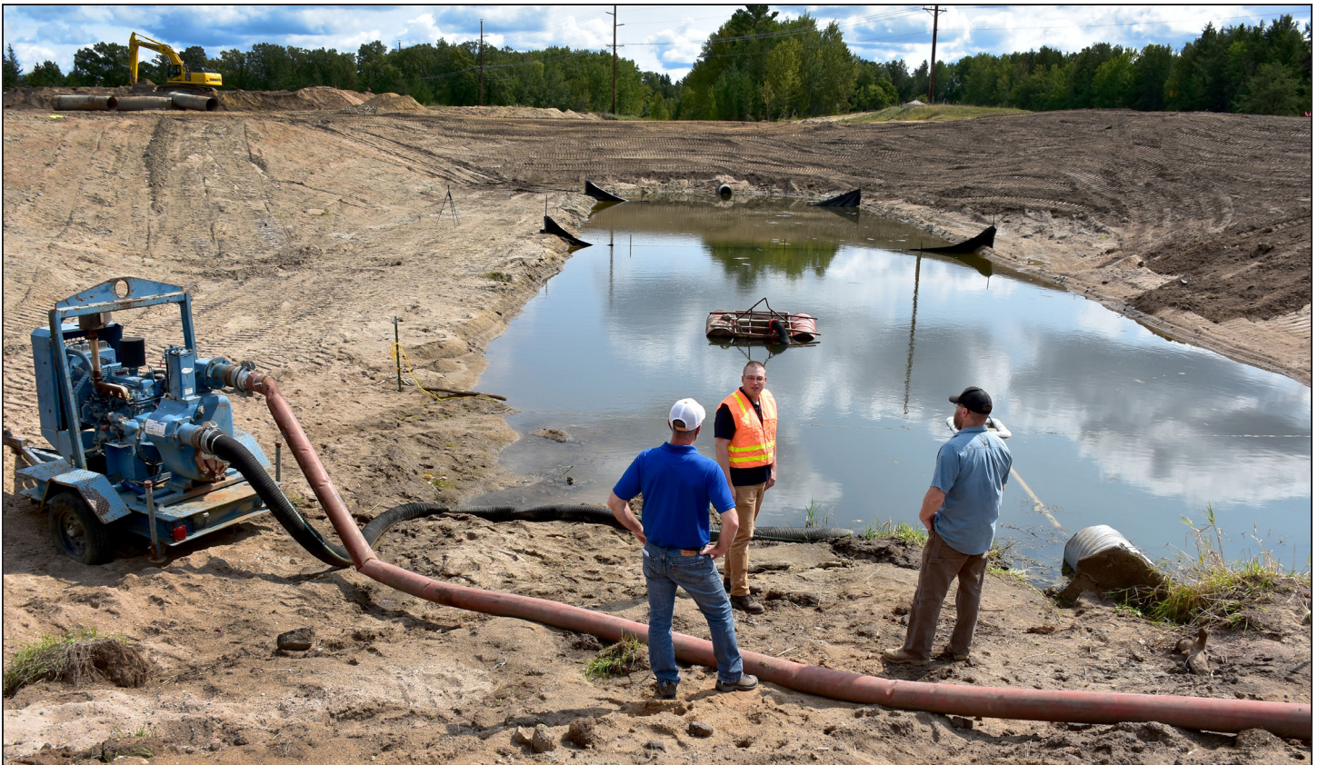
Gutknecht, center, visited the construction site of a stormwater treatment project Sept. 9, 2021, in Bemidji with Tracy, right, and Severts. An iron enhanced sand filter is part of the Clean Water Fund-backed stormwater project designed to improve the water quality of nutrient-impaired Lake Irving. The Mississippi River connects Lake Irving to Lake Bemidji; the project also will protect Lake Bemidji's water quality. The work will keep an estimated 233 pounds of phosphorus out of Lake Irving each year.
