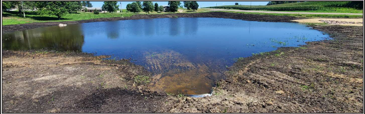
Contractors in summer 2020 excavated more of the wetland to increase flood storage, and installed a culvert connecting it to the upper watershed. Photo Credit: Le Sueur County SWCD
