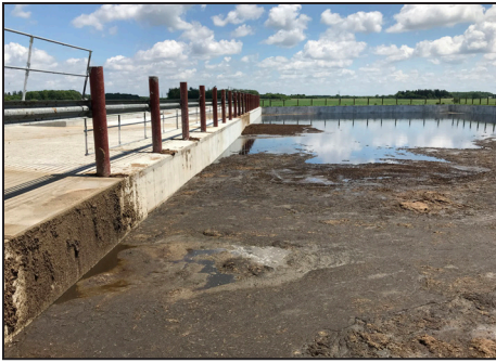
Left: The fencing Ben and Jay Currier installed along the edge of the pit can be raised and lowered. Having two points to scrape manure into the pit gives them an option if buildup occurs during winter freezes. The 1.4 million-gallon design allows for increased volume due to rainfall. Middle: The previous storage area, left of the open barn door, held a week's worth of manure. Right: A ramp makes clean-out easier.
