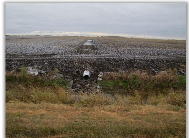
Side Water Inlet (SWI) installed with state funds
