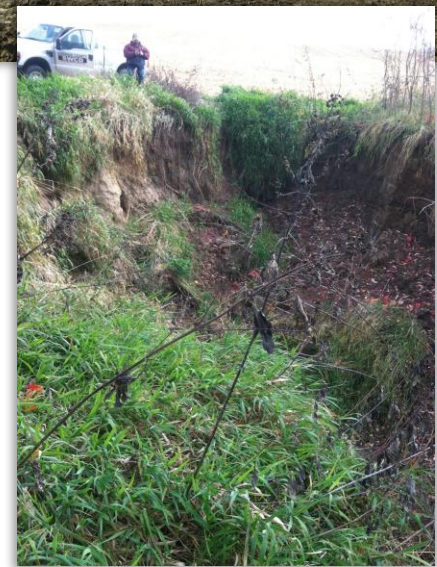
A water and sediment basin is installed on a local property.
