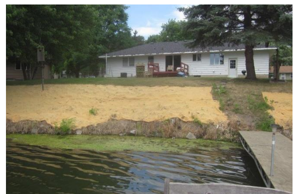
A shoreline restoration project in Scott County..
