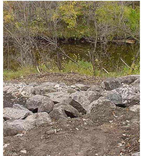
A streambank stabilization project on the Roseau River.
