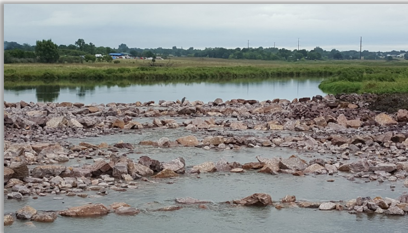
Indian Lake dam replacement
