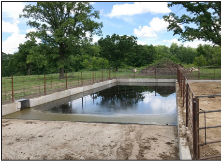
Left: Solids settle and water evaporates from a basin. The remaining water travels through tile to a vegetated treatment area, where solids settle out as the water flows across a series of alternating gravel and grass strips on its way to a grassed waterway. Middle: A covered-roof stacking slab provides six months of manure storage. The 50-by-80-foot building has 4-foot-tall concrete walls and an attached, uncovered area. Right: Fencing will allow rotational grazing paddocks within the 10-acre pasture in Mayhew Lake Township.
