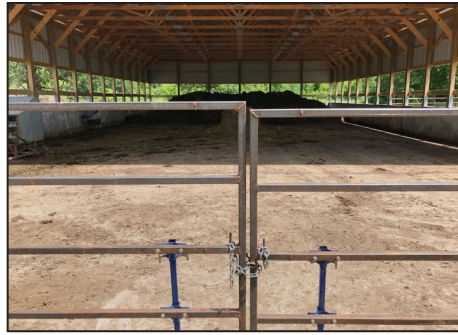
Left: Solids settle and water evaporates from a basin. The remaining water travels through tile to a vegetated treatment area, where solids settle out as the water flows across a series of alternating gravel and grass strips on its way to a grassed waterway. Middle: A covered-roof stacking slab provides six months of manure storage. The 50-by-80-foot building has 4-foot-tall concrete walls and an attached, uncovered area. Right: Fencing will allow rotational grazing paddocks within the 10-acre pasture in Mayhew Lake Township.
