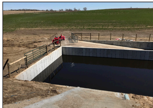
An earthen berm surrounds the concrete lagoon. An emergency spillway opens to a meadow. Manure from the dairy barn and heifer lot, above, is scraped into the lagoon.
