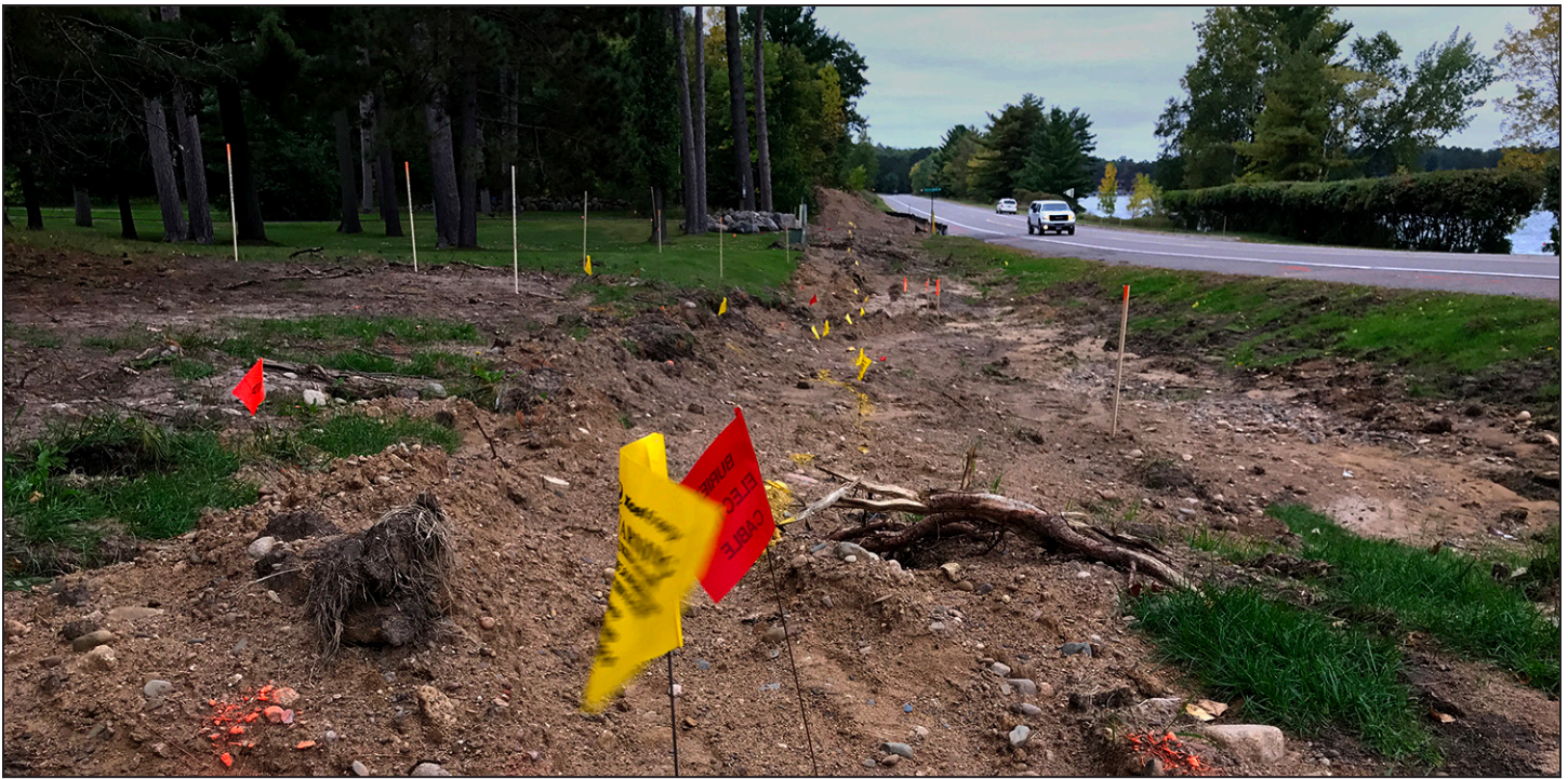
Crow Wing County Road 66 parallels Big Trout Lake just outside Manhattan Beach. A Crow Wing Soil & Water Conservation project will treat stormwater runoff that enters the lake here. The project is designed to treat a 1-inch rain and projected to keep 40 tons of sediment and 40 pounds of phosphorus out of the lake annually.
