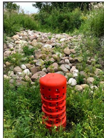
Top: Before the nine side-inlet control structures were installed, the lateral feeding County Ditch 8 drew thrill-seekers with big pickups with mud tires. Each culvert was sized to fit the area affected. Bottom: A perforated, above-ground inlet pipe provides another release for backed-up water at locations where water is meant to stand for a short time, allowing sediment to settle out. Photo Credits: Ann Wessel, BWSR
