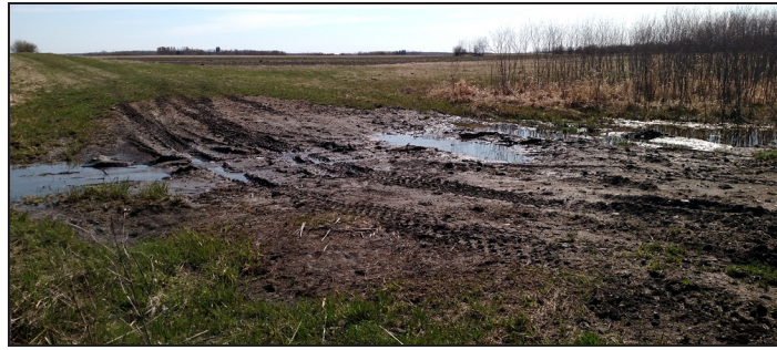
In wet conditions, this minimum-maintenance road was nearly impassable. The road had been cut in low, swampy spots. It drew big trucks with mud tires. Photo Credit: Roseau River Watershed District
