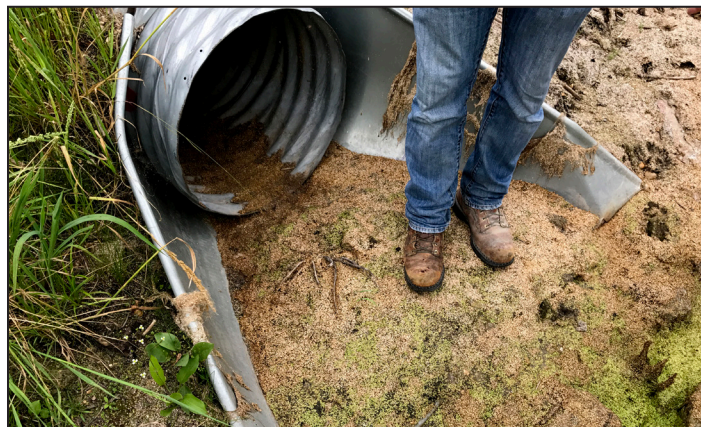
Top: Nine side-inlet control structures were installed in fall 2016 where a lateral feeding County Ditch 8 runs parallel to a mile-long stretch of minimum maintenance road. Crushed asphalt tops the road where culverts were installed. The road slices through long, linear wetlands. Bottom: Once fixes are made farther up in the watershed, the culverts will be cleared of excess sediment. Photo Credits: Ann Wessel, BWSR
