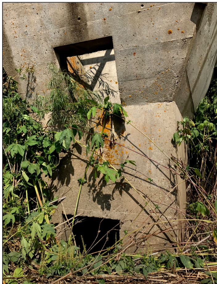
After 60 years, sediment was flush with the lower inlet. In recent years, the 3-acre settling pond was farmed.
