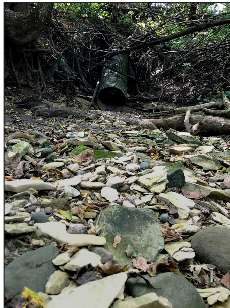
Above: A failing culvert at the edge of Pederson's corn field was on the brink of washing out in September 2017. It was replaced, and the channel was stabilized. The ravine leads to the Cedar River. Below: The view of the culvert from the ravine looking toward the corn field shows the path runoff followed to Cedar Creek south of Austin.
