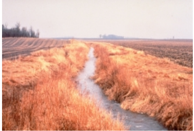
Figure 6 – Typical Drainage Ditch for Southern and Western Minnesota with Narrow Grass Buffer Strips - Fall
