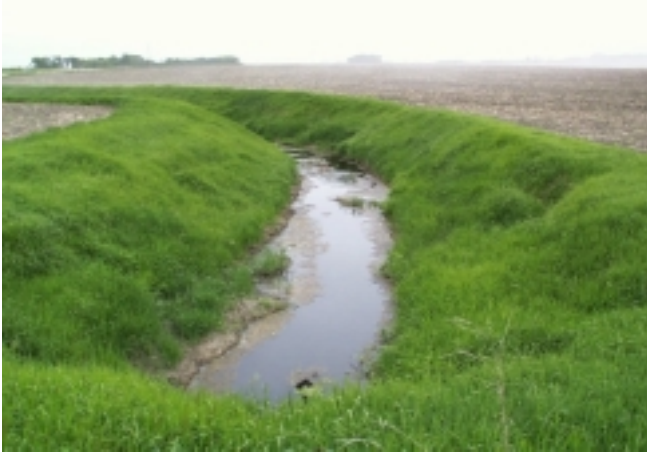
Figure 5 – Typical Drainage Ditch for Southern and Western Minnesota with Narrow Grass Buffer Strips - Spring
