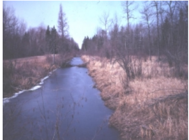
Figure 10 – Example of Drainage Ditch in Northern Minnesota
