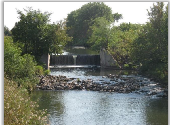
One of the Army Corps drop structures installed between Fertile and Beltrami, Minnesota on the Sand Hill River. This structure will be modified as part of the project.
