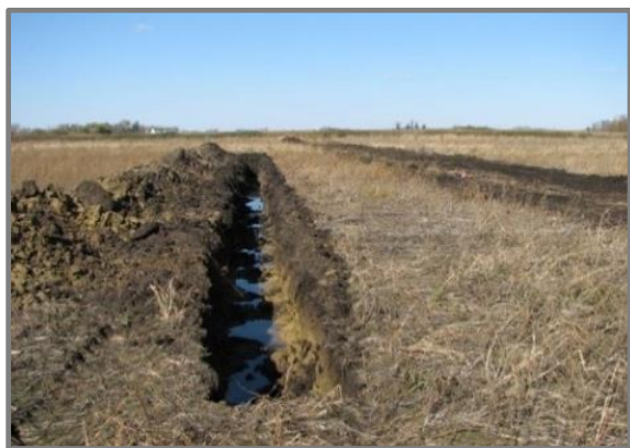
Figure 12. Tile Investigation Trench
