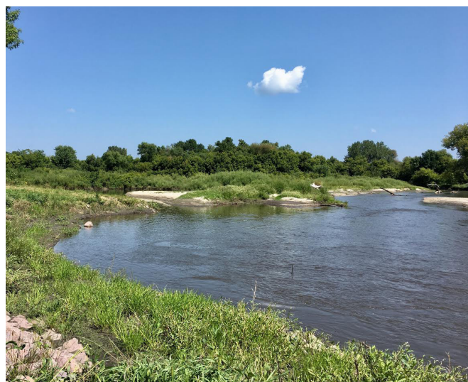
One tour stop showed a stream bank restoration site along the Rock River in Luverne. The project prevented the stream from cutting a path through an old landfill site after severe flooding in 2014.
