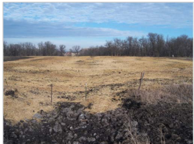
Grassed waterway and drop structure completed in 2012.
